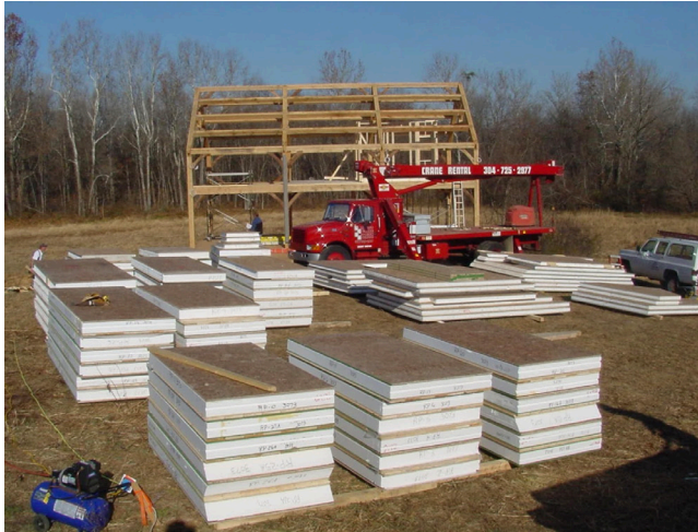
IMAGE 5.6: SIPS STAGED ON JOBSITE
