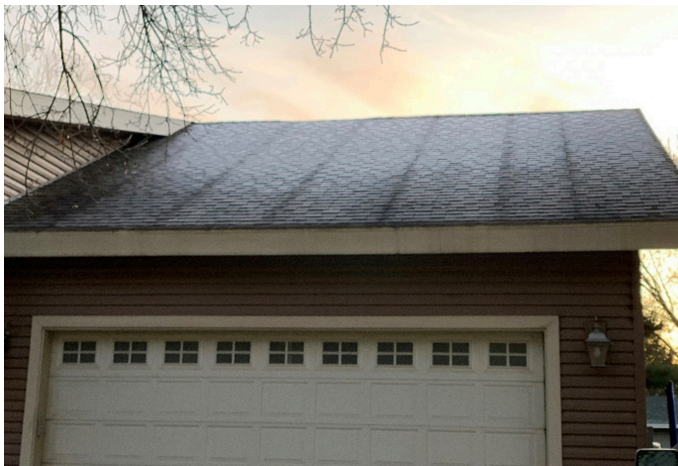
IMAGE 1.3: SIP GARAGE ROOF
