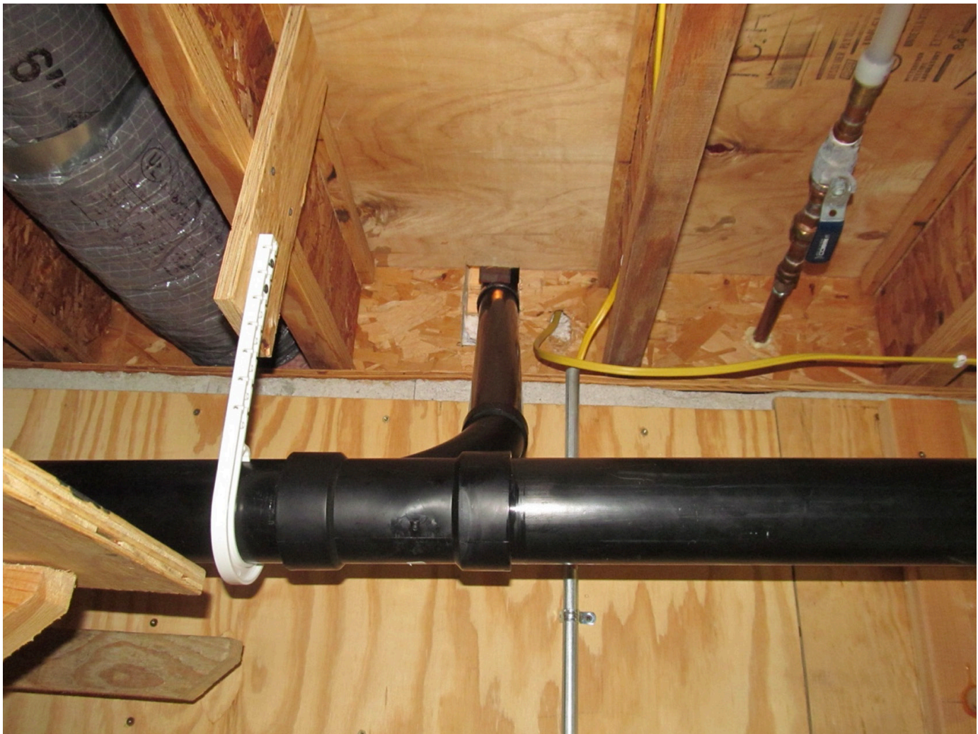
IMAGE 10.1 PLUMBING VENT PIPE GOING INTO SIP WALL
