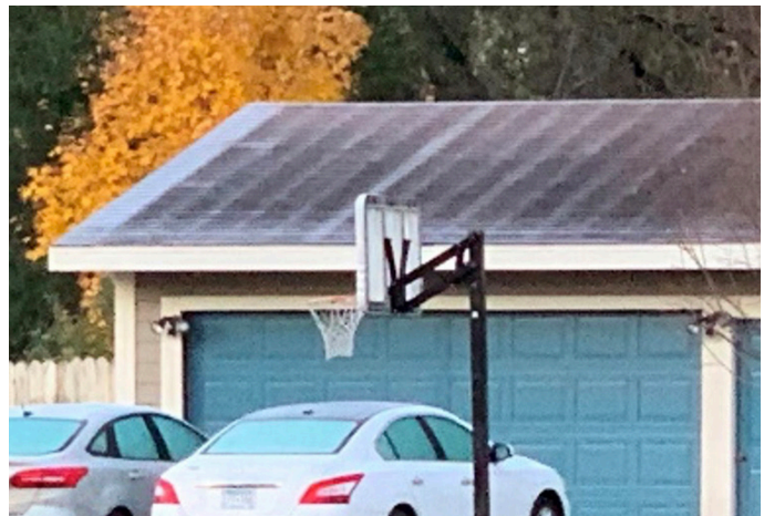
IMAGE 1.4: TRADITIONAL GARAGE ROOF
